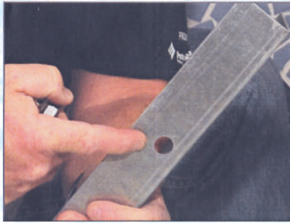
1 - The pre-punched hole in the short angle for clip to be applied
