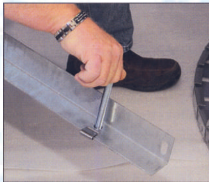
3 - The bolt is installed through pre-punched hole and clip
